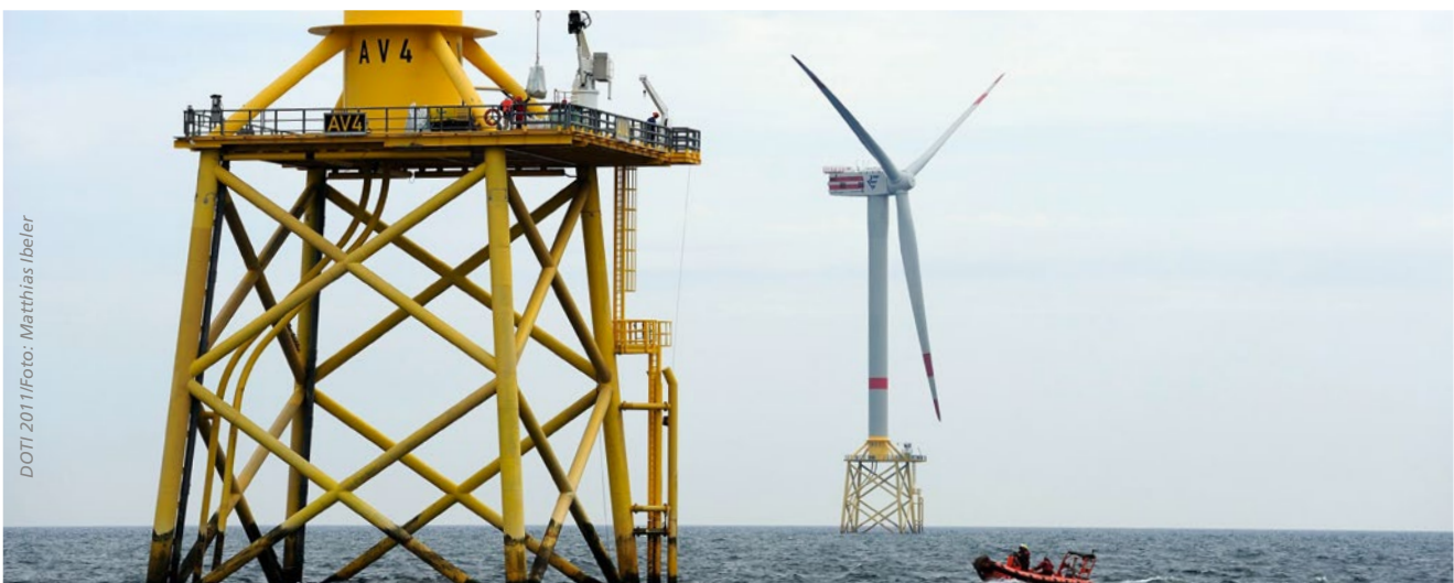
Jacket foundation of the „alpha-ventus“ wind farm
